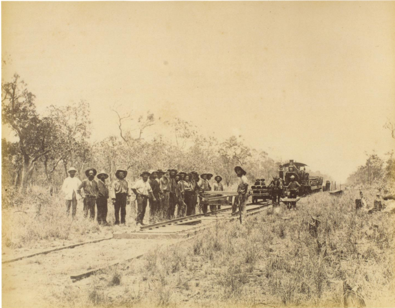
Head of road at 25½ miles: Plate laying gang.
