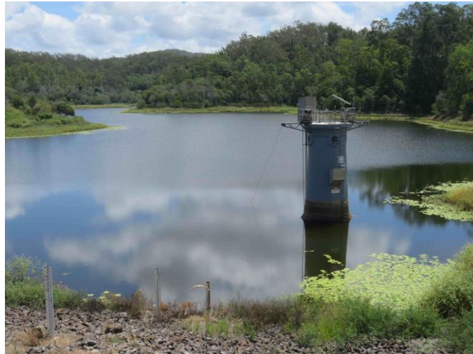
Gold Creek Reservoir water intake; credit Ralph Carlisle
